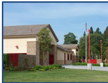
Figure 1 Pinehurst Fire Station
